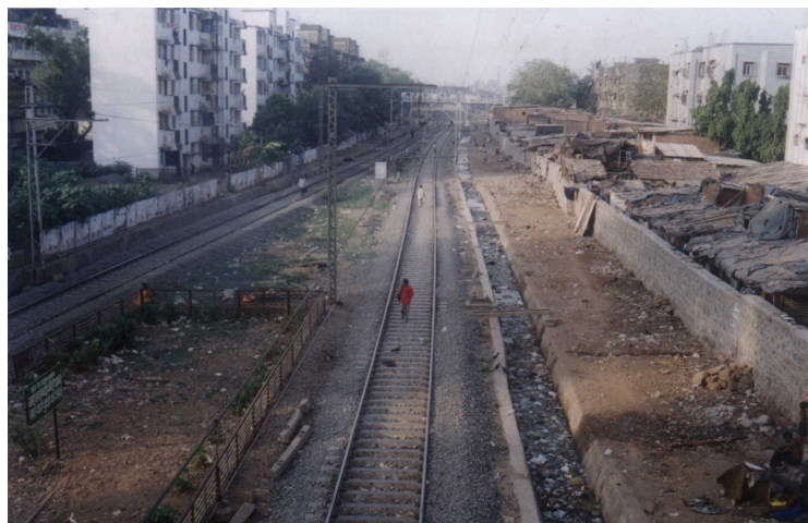
Land adjacent to the tracks cleared of encroachments to create a ten meter Safety Zone. (Photo Credit: SP-ARC)
